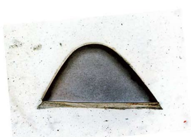
Photos: HT Consultants
